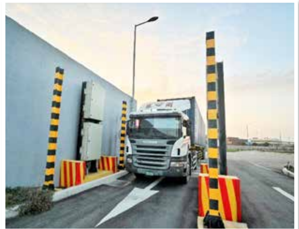
貨櫃輻射安全偵檢 Container Radiation Security Detection
