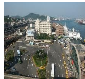
Photo 2: Harbor Building is located at the metropolis Centre.
