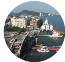
Photo 1: Harbor Building is located at the metropolis Centre.
